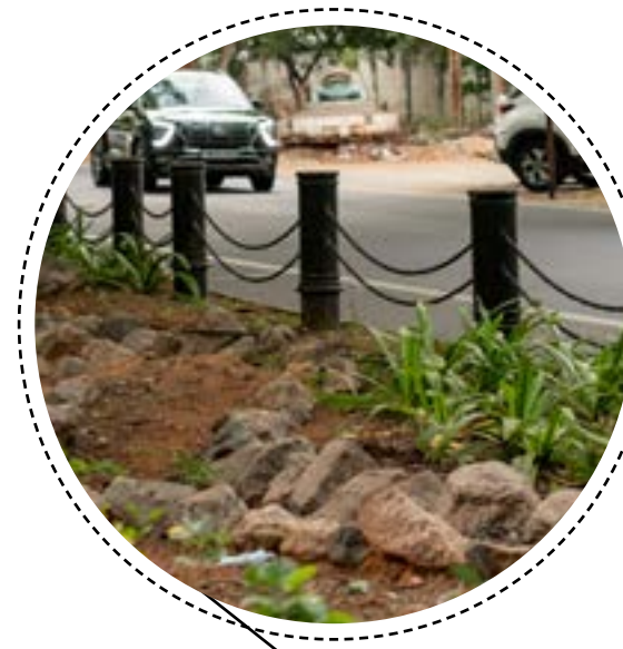
Stormwater swale within the landscape zone
